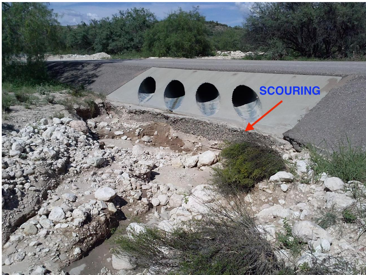
Figure 1.4: Pipes Exit with some scour forming
