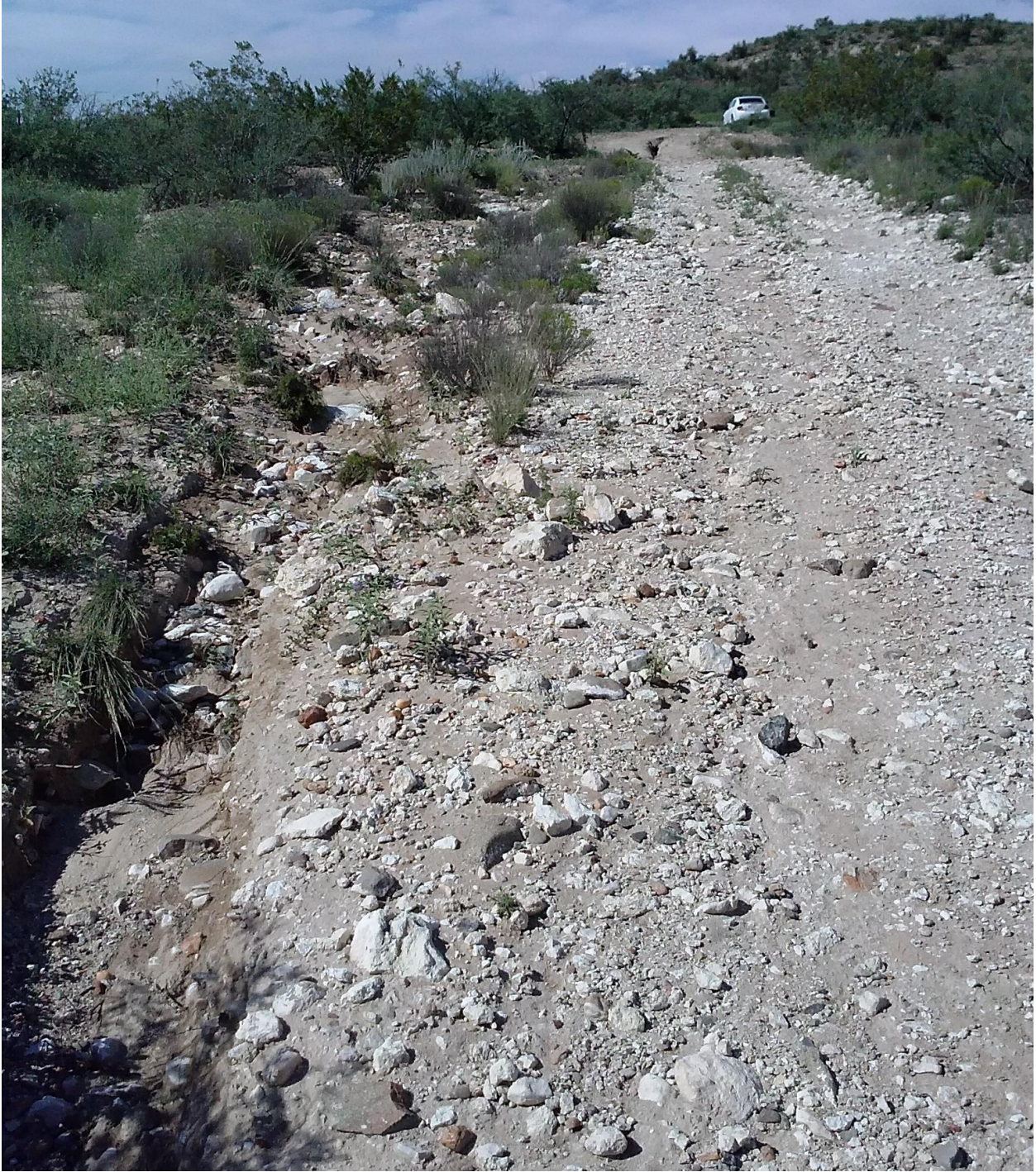
Figure 1.5: Existing Dirt Road Conditions: Drainage on side of road
